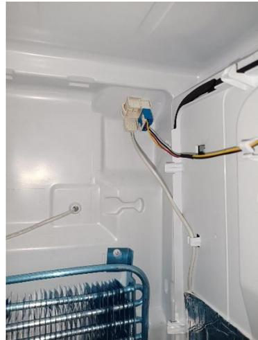
**Fan motor of air duct**
