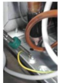
Finally, the inverter is released by disconnecting the ground wire
